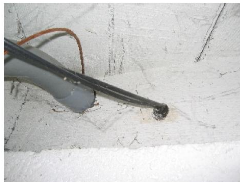
Air leakage through holes in basement rim joist.
