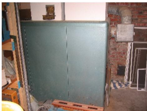
Oil converted to gas furnace.
