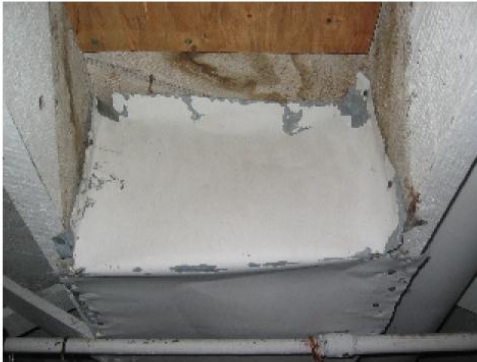
Leaky panned joist duct.
