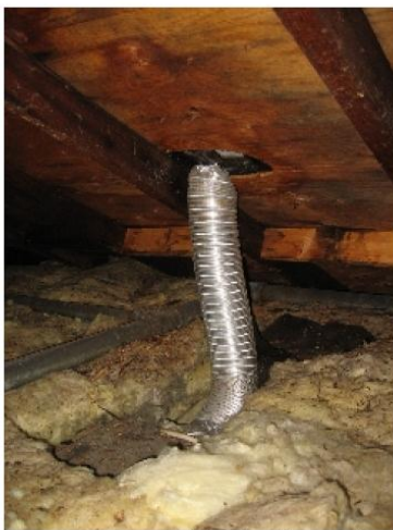
Bath fan ducted improperly to roof vent.
