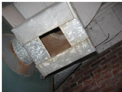
Furnace draft hood: exhaust gases inside.
